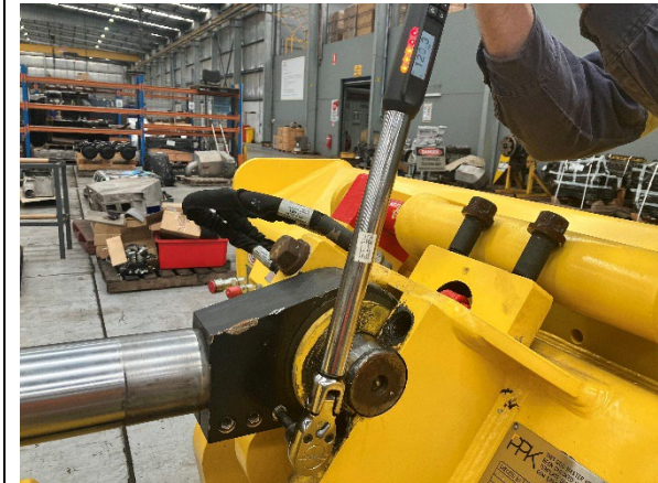
Figure 8. Tension new bolt to the recommended torque of 120 Nm.
