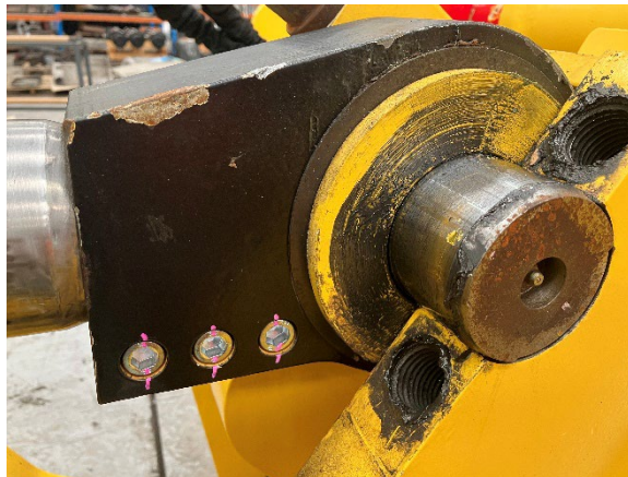
Figure 10. Mark each bolt head corresponding with the clevis body on completion of bolt torque sequence.
