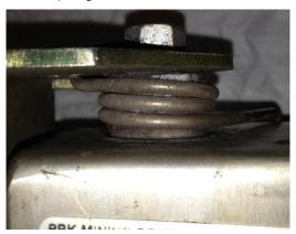
Figure 1: Old spring with 2 full coils (3 visible strands)
