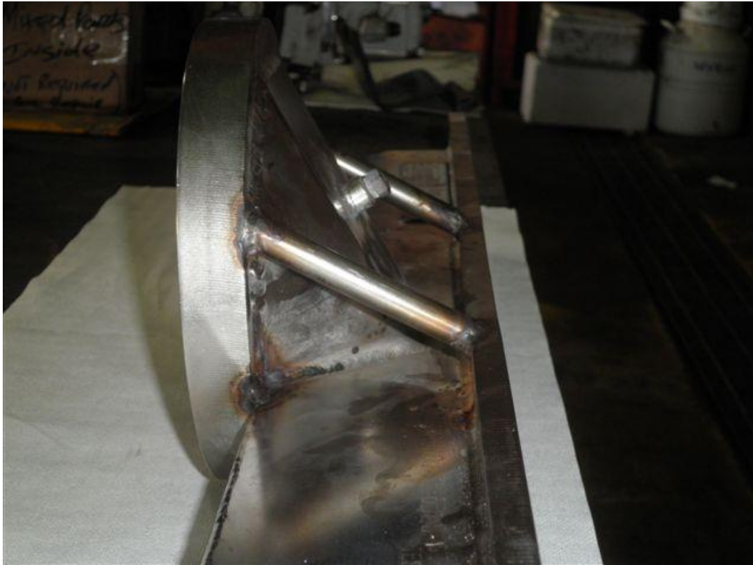
Figure 3: Photograph showing the additional supporting braces added to the exterior of the inlet manifold for additional support for the flametrap housing.
