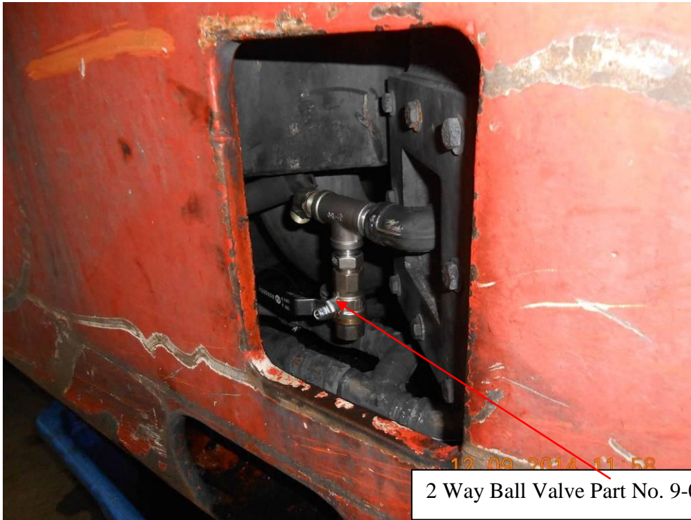
Figure 1: New 2 Way Low Water Test Valve Installation.
