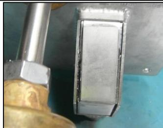
Float Sensor with blanking plate over indicator lights
